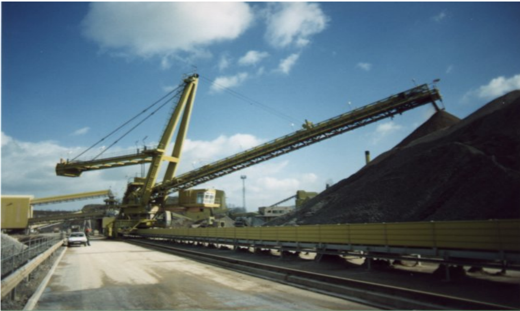
Typical dynamic test of a material conveyor system in a quarry
